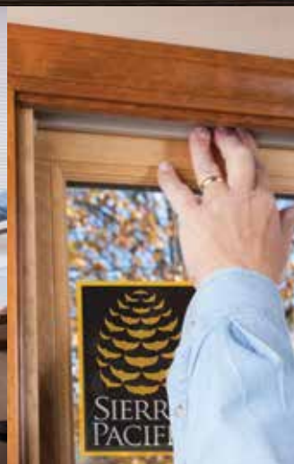
Step 4 Install new head weatherstripping.
