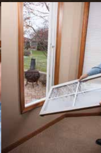
Step 3 Install new sash.
